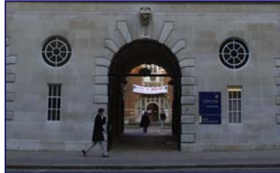
Imperial College London Beit Halls of Residence Prince Consort Road London SW7 2AZ
