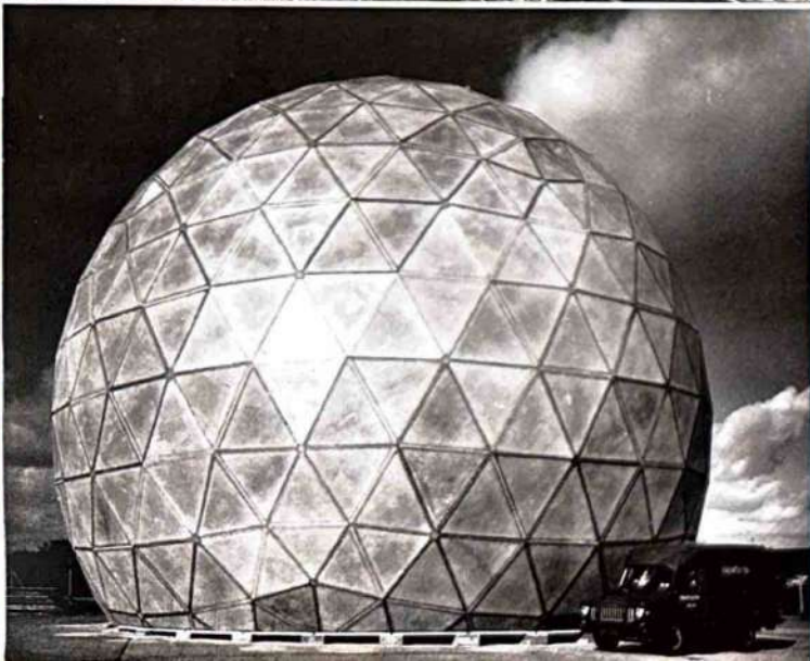
One of the many new applications of reinforced plastics – an English Electric radome for the protection of defence radar equipment
