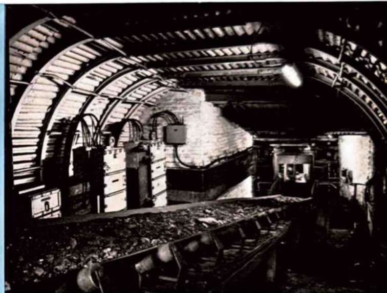
Automatic coal-handling system controlled by English Electric static switching equipment
