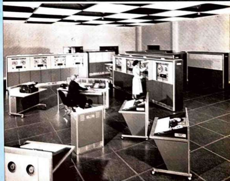
A KDP10 data-processing system dealing with the records of five million insurance policy holders, reviewing and bringing up to date as required 1½ million policies per day
